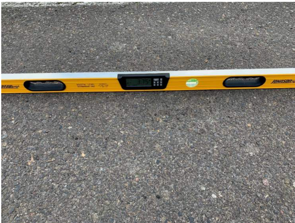
Photo 5—Approx 3.8% slope to south in parking lot from Photo 4 above.
